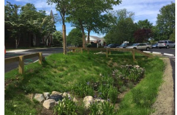
Bioretention Area – Parking Lot Public Library, Sandwich, MA
